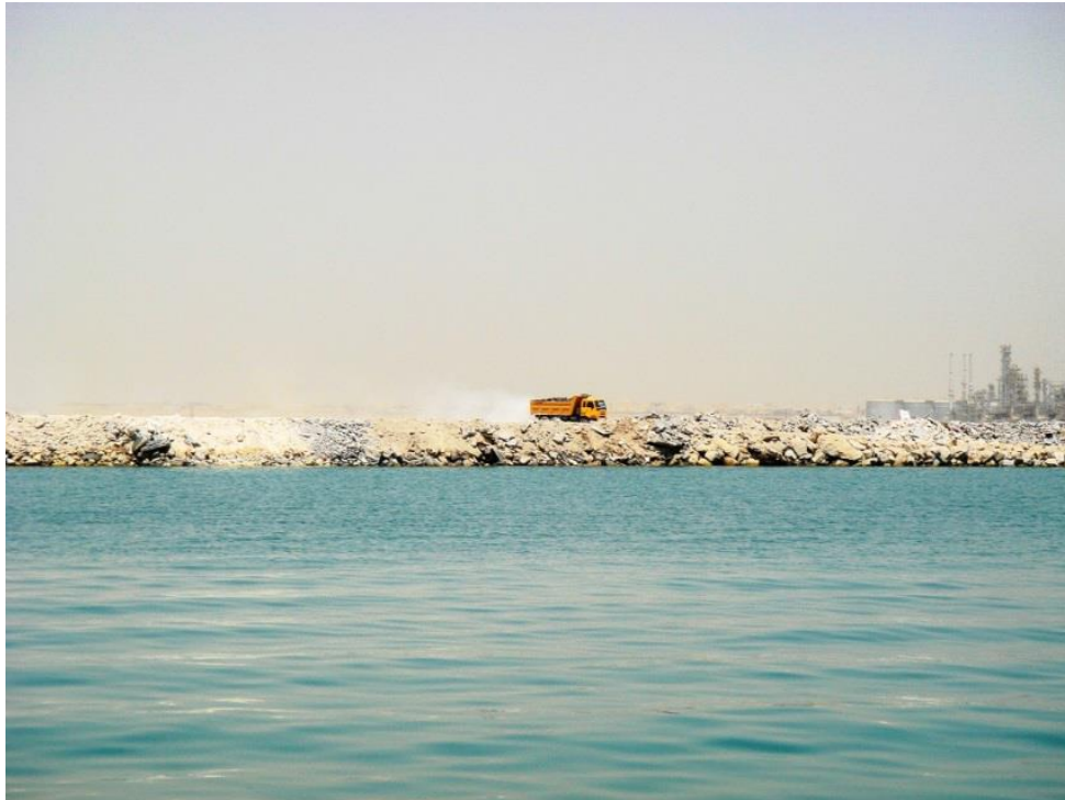
Figure 12. Rocks and sands extracted from nearby quarries are used to reclaim a coastal area along the eastern coastline of Bahrain-2012 (Naser, 2014).
